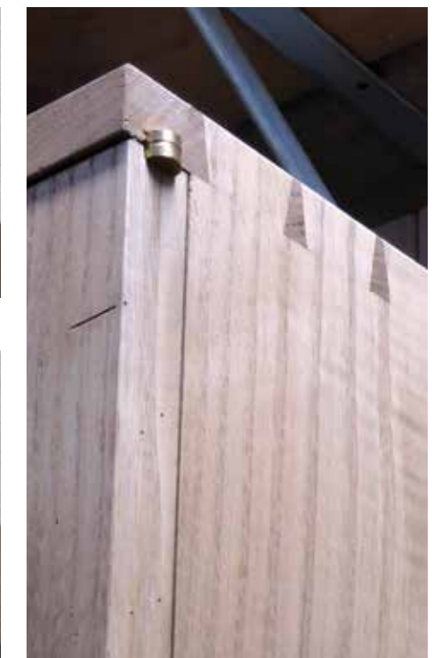
Just the knuckle is exposed at the side of the cabinet
